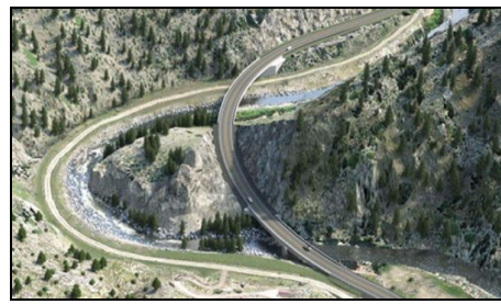
Post-flood bridge repair at Horseshoe Curve, Big Thompson River. This part of Highway 34 was washed out in the 1976 and 2013 floods. (Photo: Kiewit Infrastructure Company )
