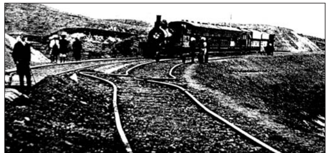
Plate 6 Contraction of the railway line where it crossed the 1892 Chaman fault (from Griesbach 1893). Sinistral fault slip is estimated here to have exceeded 70 cm.
