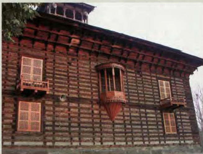
Figure 3. Traditional construction in Kashmir incorporated a mixture of timber and masonry elements. Referred to as dhajji-dewari , this system served not only to make the best use of available local materials but also proves to be very robust in an earthquake. These buildings in Srinagar, Kashmir, are tied together by wooden posts and beams and have masonry infill. Note also the metal tie straps at the building corner in the right-hand photograph. Unfortunately, as the population of Kashmir has surged to five million in recent years, new construction has abandoned the time-tested techniques in favor of a ramshackle hodgepodge of masonry buildings with little resistance to ground shaking. (Photographs by Roger Bilham unless otherwise noted.)
