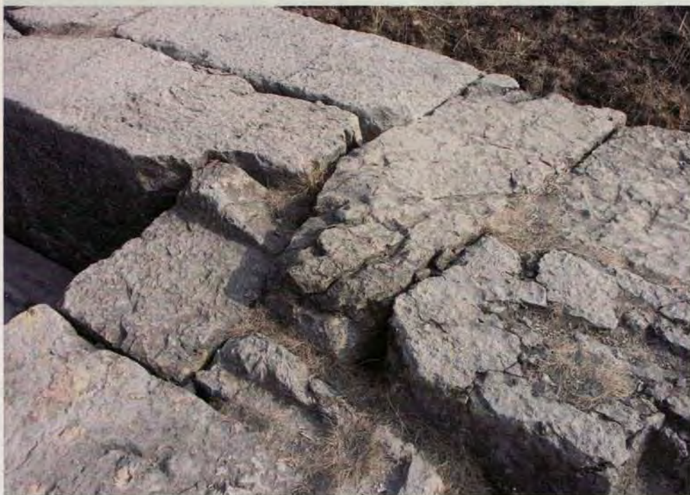
Figure 7. Martanda Sun Temple has been spared the full ravages of not only Sicuter the Iconoclast, who razed many temples in Kashmir, but also the shaking of many large earthquakes. The authors attribute the temple's seismic survival to two important features. First, the temple was built about 90 meters above the valley floor on competent rock not subject to amplification of motion by unconsolidated sediments. Second, the masonry construction incorporates massive carved interlocking stone blocks fitted tightly together.
