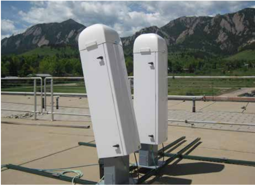
GMD-01: Two Vaisala Model CL51 Ceilometers installed on the NOAA David Skaggs Research Center roof in Boulder, Colorado. Units are being tested before permanent field deployment. In order to test side-by-side, one unit is tilted slightly so the retrieved signals do not interfere with each other. Photo: Gary Hodges/CIRES
