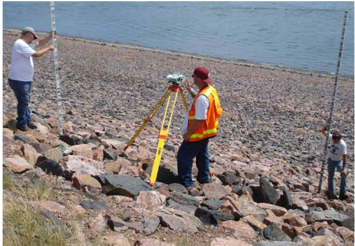
Field surveyors Nick Michael, Dave Salter and Michael Swinford run a level loop to establish current year elevations for tiltmeters, sensitive inclinometers designed to measure small structure changes, at Cherry Creek Dam near Denver, Colorado. Photo: U.S. Army Corps of Engineers
